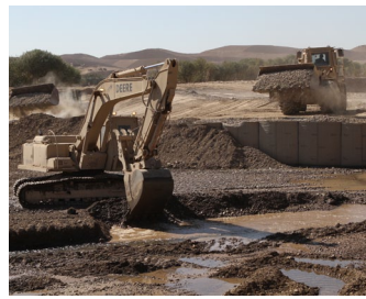
Redirecting stream & filling Hescos
