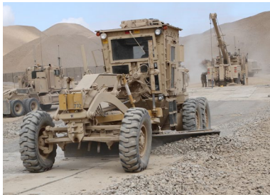
Grader spreads out gravel.
