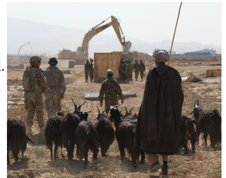
Project nears completion as shepherd passes by
