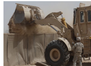
Loader filling in Hesco wall.
