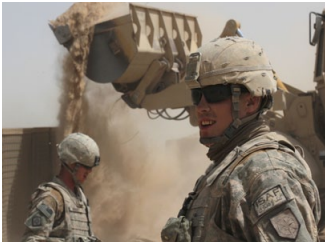
SGT Nicholas McElroy w/ Det.1, 623rd EN CO looks at the completed HLZ wall.
