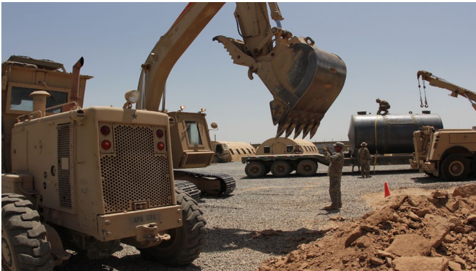
Construction site at Combat Outpost Shir Khan.
