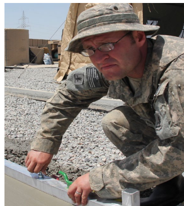
SPC Foster tightens forms for cement
